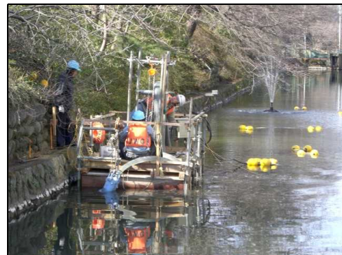
Sludge is mixed by an agitation pump on dredger. High concentration of mud water is sucked by a dredging pump.
