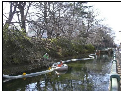
Mud water is sent to a treatment plant through pipes, to correspond with the movement of the dredger, we set up pipes with floats on the water and set up laying metallic pipes on the ground.
