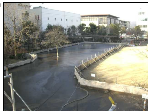
Muddy water which MSC agitated is released to a treatment yard and separates hydrophobicity immediately. There is no offensive odor during construction with the odorless function of MSC.
